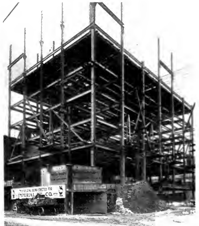
Steel erection, March 21, 1916.
